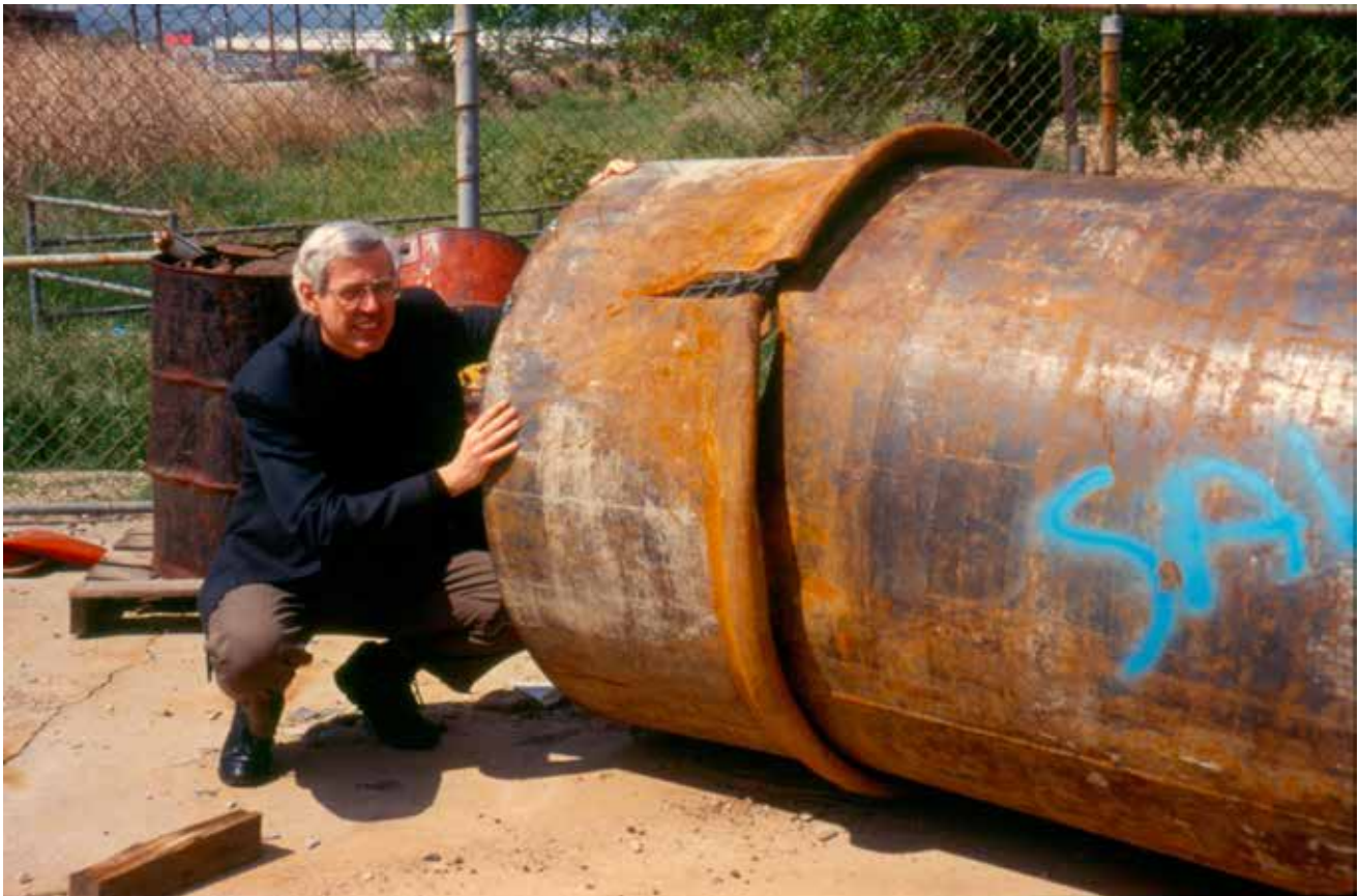
Examining the damaged Granada Trunk Line after the 1994 Northridge earthquake in the San Fernando Valley in California.
