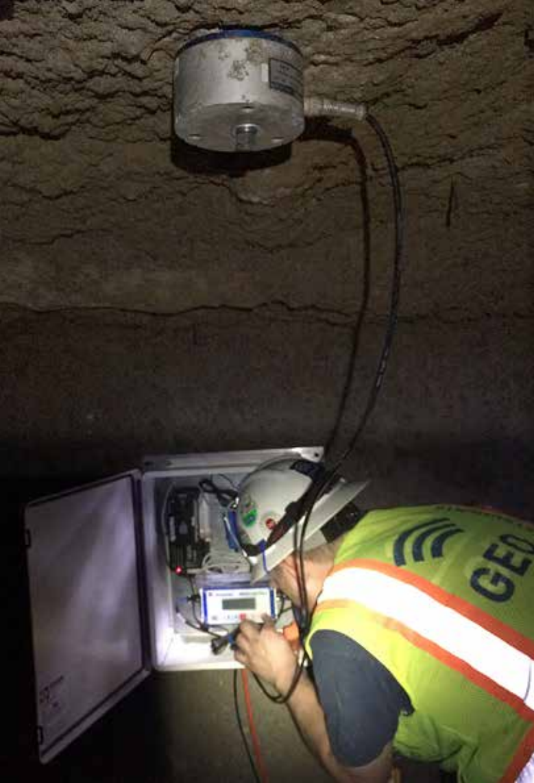
Figure 5. Automated vibration monitoring of Metro tunnel while construction occurs nearby.
